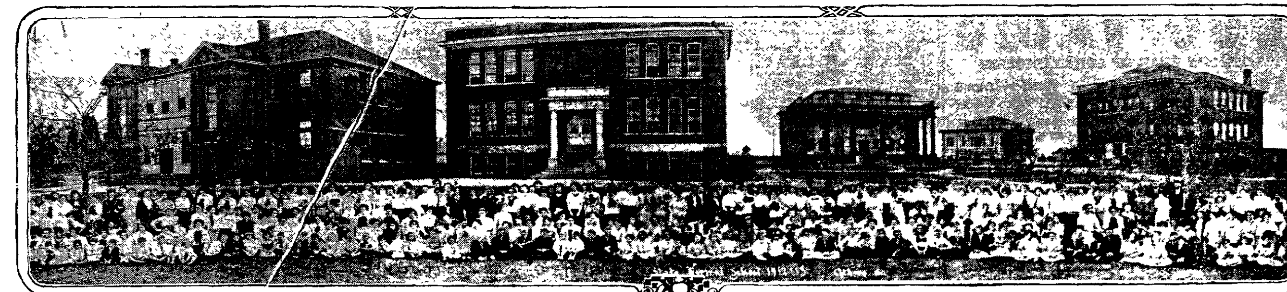
State Normal school grounds and part of this year's student body. The buildings, from left to right, are: President's cottage, auditorium, James Smith building, Winnie Davis hall, library, country school (small house), Muscogee practice school, and the dairy barn.
